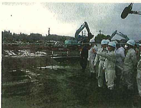
(益城町既存仮置場)
