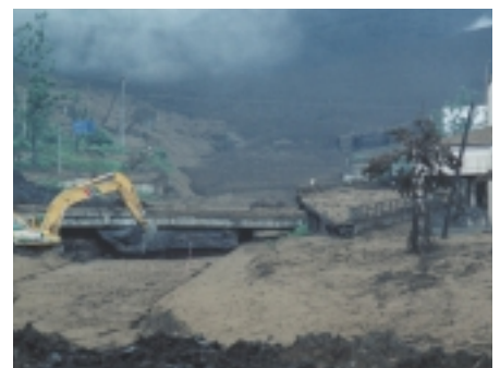
Restoration Work at Mt.Usu under Remote Control
