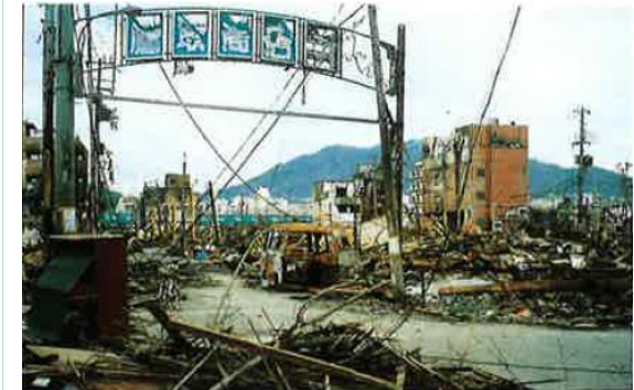
Takatori Shopping Street immediately after the Earthquake (1995)
