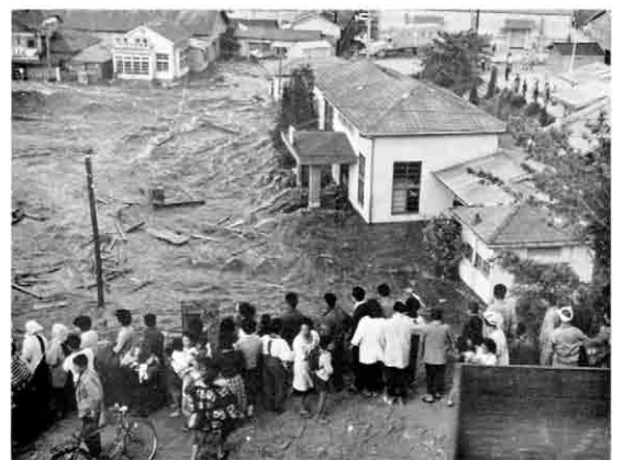
g. 29. Flooding by the fourth wave of the Tsunami at Onagawa Railway Station, Miyagi Pref. at 4h 45 m, May 24. (Photo taken by M. Kondō.)
