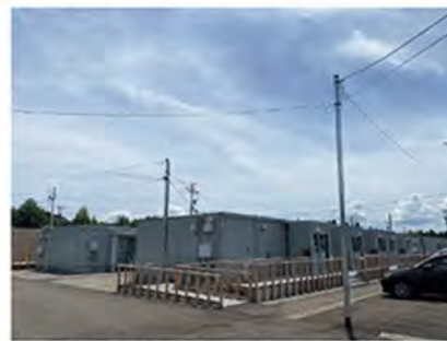
Prefabricated emergency temporary housing
