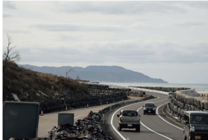
A detour route utilizing the uplifted coastline (near Shirome Senmaida, National Route 249)
