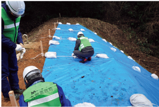
MAFF-SAT installs blue tarps on damaged reservoir (Shika Town)
