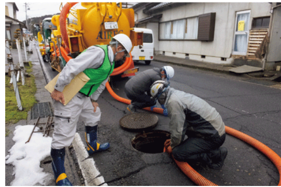
Inspection of agricultural village drainage facilities using MAFF-SAT (Noto Town)
