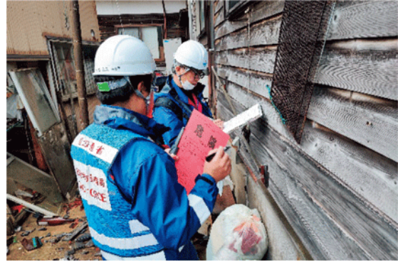
TEC-FORCE filling out and attaching assessment stickers (Anamizu Town)
