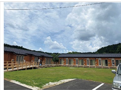
Temporary housing complex made of wood
