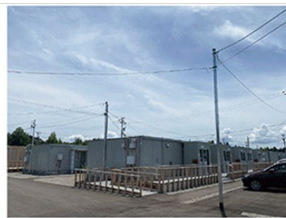
Prefabricated emergency temporary housing
