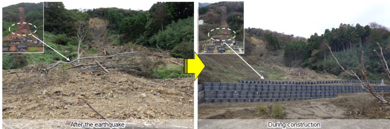
Forest under construction as part of a disaster restoration project (Oya-cho, Suzu City, Ishikawa Prefecture)
