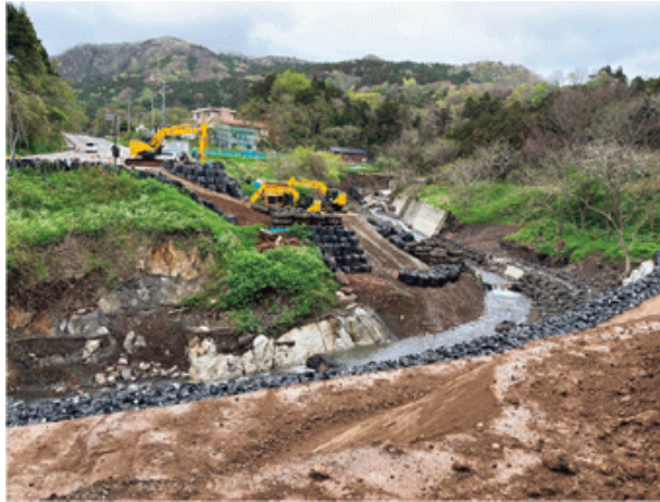
Construction of landslide prevention work under delegated authority (Wajima City, Ishikawa Prefecture)
