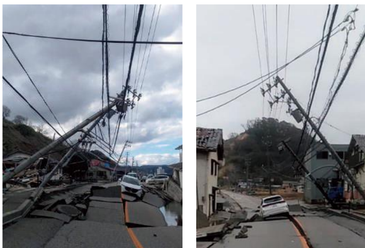
Utility poles that collapsed due to the earthquake Source: Hokuriku Electric Power Transmission & Distribution Company
