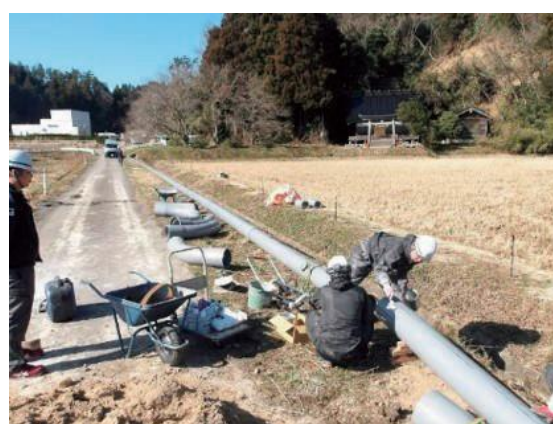
Laying of temporary pressure feed pipes in Suzu City Source: Ministry of Land, Infrastructure, Transport and Tourism (MLIT)
