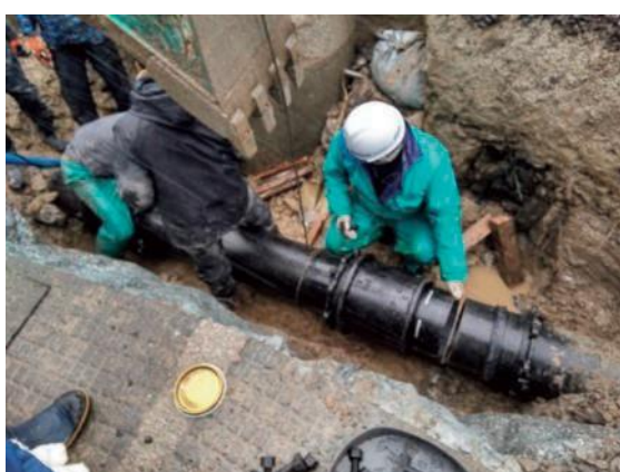
Restoration of water supply pipes in Wajima City Source: Ministry of Land, Infrastructure, Transport and Tourism (MLIT)
