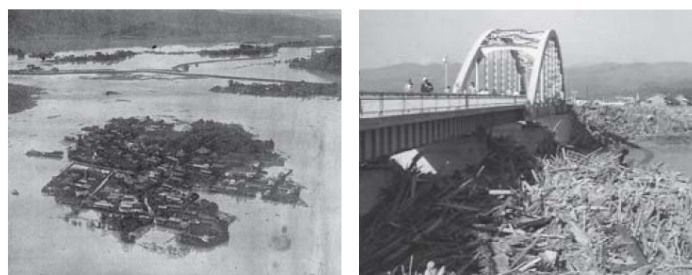
Photo 7. Damage Caused by Kanogawa Typhoon in September 1958
