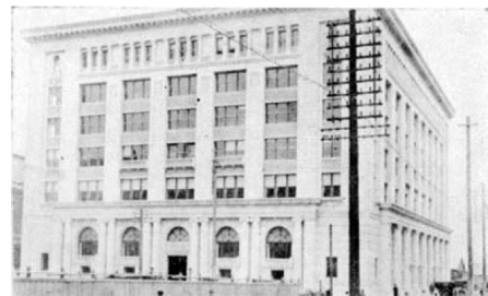
Industrial Bank of Japan (It was completed in 1923 and designed by Tachu Naito, incorporating earthquake-resistant walls.)
