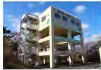
Evacuation tower with a cold-weather protection function
