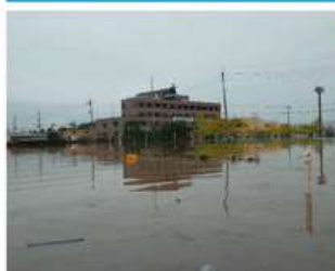
Damage at Marumori Town, Miyagi Prefecture
