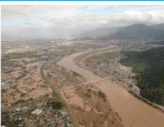
Damage at Nagano City, Nagano Prefecture
