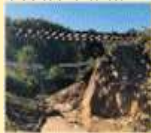
The Sanriku Railway, the erosion of ballast
