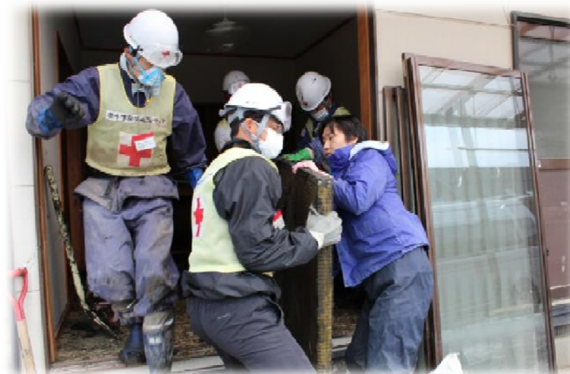
Cleaning houses flooded by tsunami
