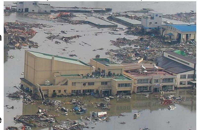
Tsunami evacuation building (Kesenuma central community center)
