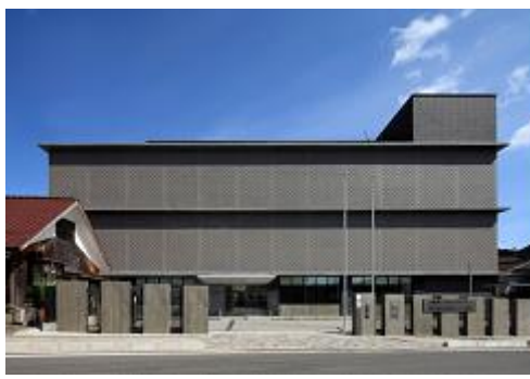
Ehime Prefecture Off-site Center
