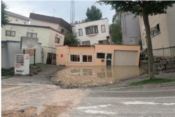
Flood due to a water pipe burst (Kiyota-ku, Sapporo City)
