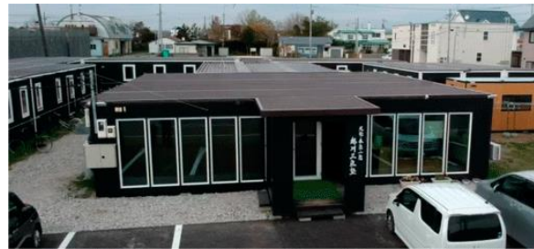
Temporary housing for students in Mukawa Town, Hokkaido Prefecture (for 36 people) Mobile houses were provided. (Photo by courtesy of Mukawa Town, Hokkaido Prefecture)
