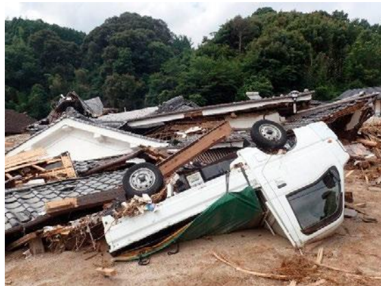
Damage due to river flooding by heavy rain (Asakura City, Fukuoka Prefecture)
