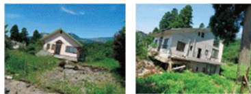
<An example of housing damage caused by slope failure in 2016 Kumamoto Earthquake>
