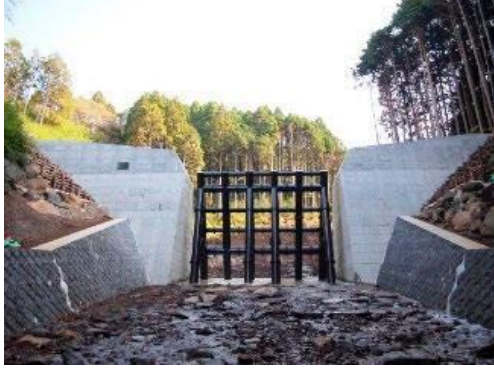
An erosion control dam of transmission type able to catch driftwood very efficiently
