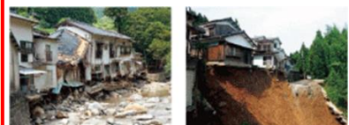
<Examples of housing damage caused by foundation and ground collapse mainly by Typhoon 18 in 2017>
