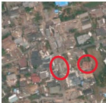
<After the 2016 Kumamoto Earthquake (taken on April 16, 2016)>
