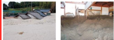
<Examples of housing damage due to sediment deposition in the 2017 Northern Kyushu Heavy Rain>
