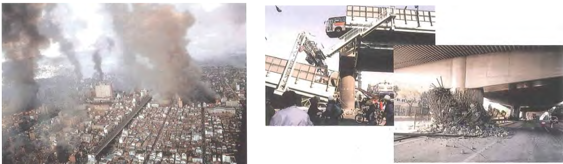
Photo 5. Damage by the Great Hanshin-Awaji Earthquake
