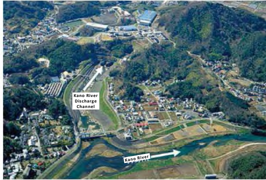
Photo 8. Kano River Discharge Channel
