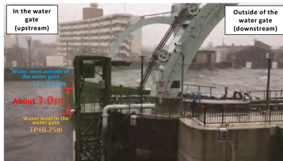
Photo 9. Kizugawa Water Gate in Osaka Bay protecting the urban area from high waves caused by Typhoon Jebi in 2018
