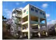
Evacuation tower with a cold-weather protection function
