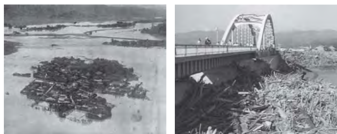
Photo 7. Damage Caused by Kanogawa Typhoon in September 1958
