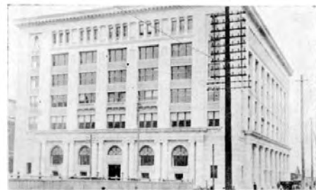
Industrial Bank of Japan (It was completed in 1923 and designed by Tachu Naito, incorporating earthquake-resistant walls.)
