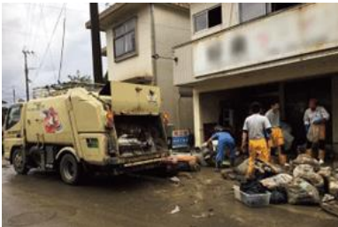
4. Clean-up operation in progress (July 12)
