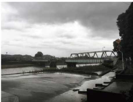
Flooding damage in Kumamoto Prefecture (Hitoyoshi City) (Cabinet Office data)
