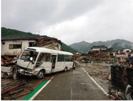
Flooding damage in Kumamoto Prefecture (Kuma Village) (Cabinet Office data)
