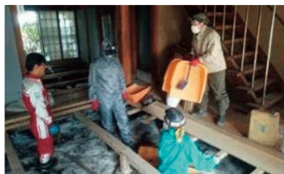
Removing mud from damaged houses
